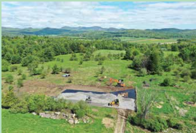
AEM project: Compost pad under construction
