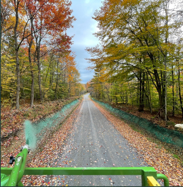
Conservation seed mix is applied to exposed ditches using a hydroseeder.
